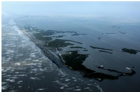
W10 Berm – November 16, 2010
