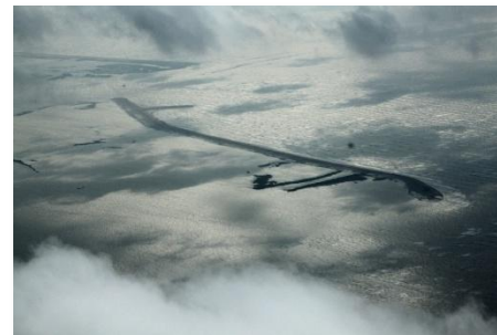
W8 Berm – November 16, 2010
