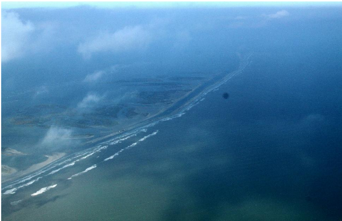
E4 North Berm – November 16, 2010
