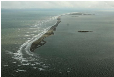
E4 Berm – November 3, 2010
