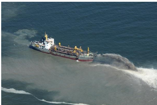
Stuyvesant Borrow Operations – September 23, 2010
