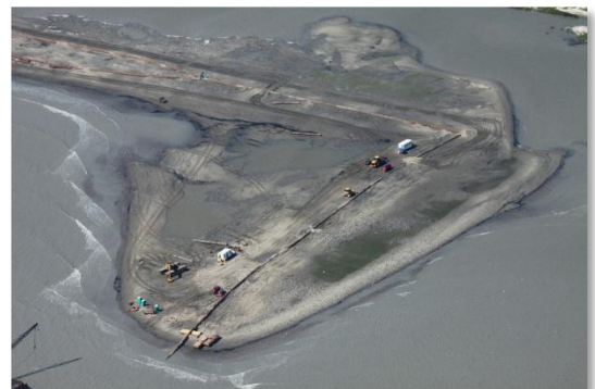
W10 Berm Operations– September 28, 2010
