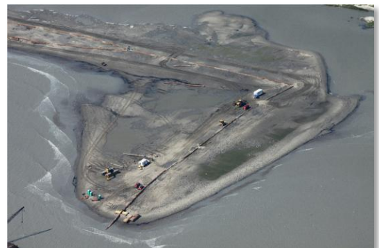
W10 Berm Operations– September 28, 2010
