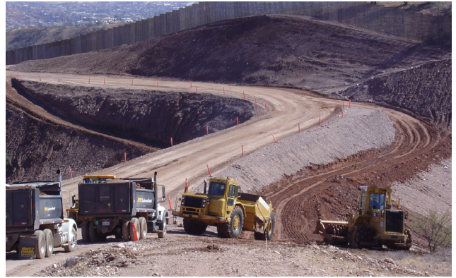
Civil Engineers support Operation Jump Start.
