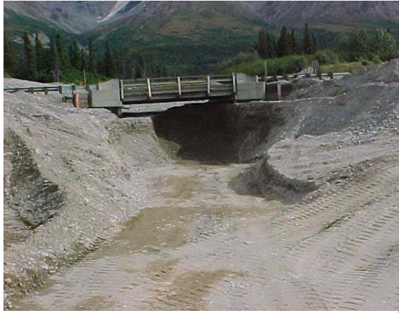
Figure 2. Photo of Richardson Highway bridge across One Mile Creek in Alaska's interior.
