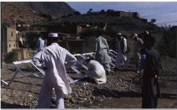
Installation Underway at Hasan Lagadai
