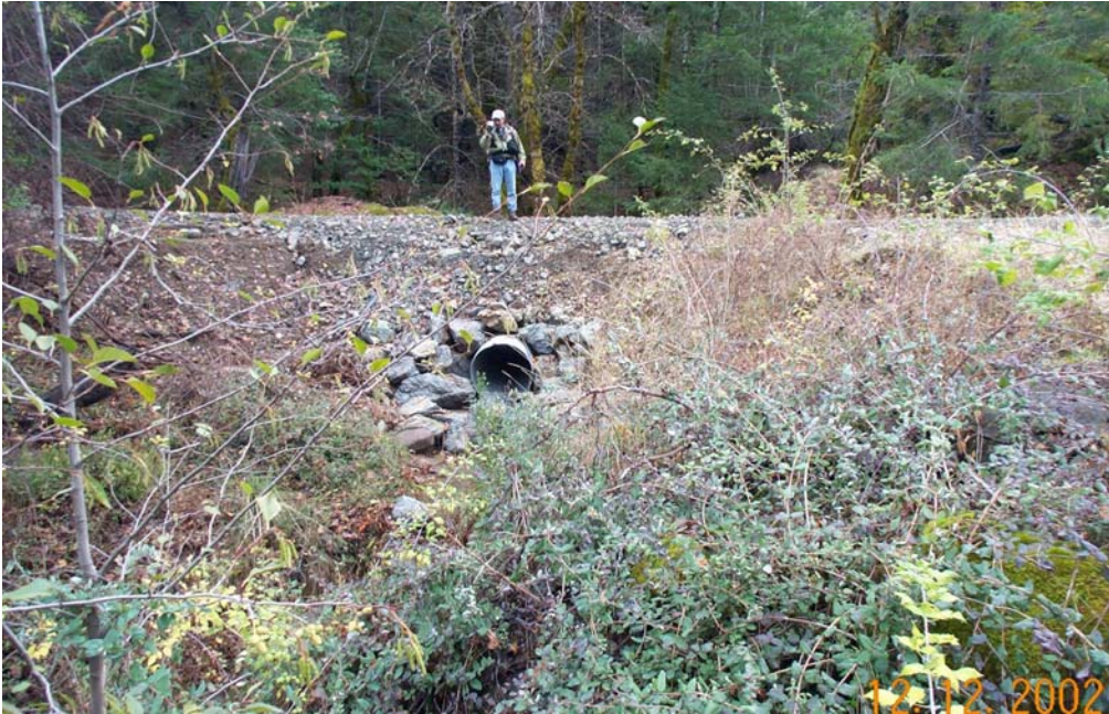
Figure 6. New culvert on tributary to lower SF Mud Springs Creek in December 2002. Tributary collects drainage from nearby fence and upslope cultivated area, and discharges into SF Mud Springs Creek at monitoring Station A.
