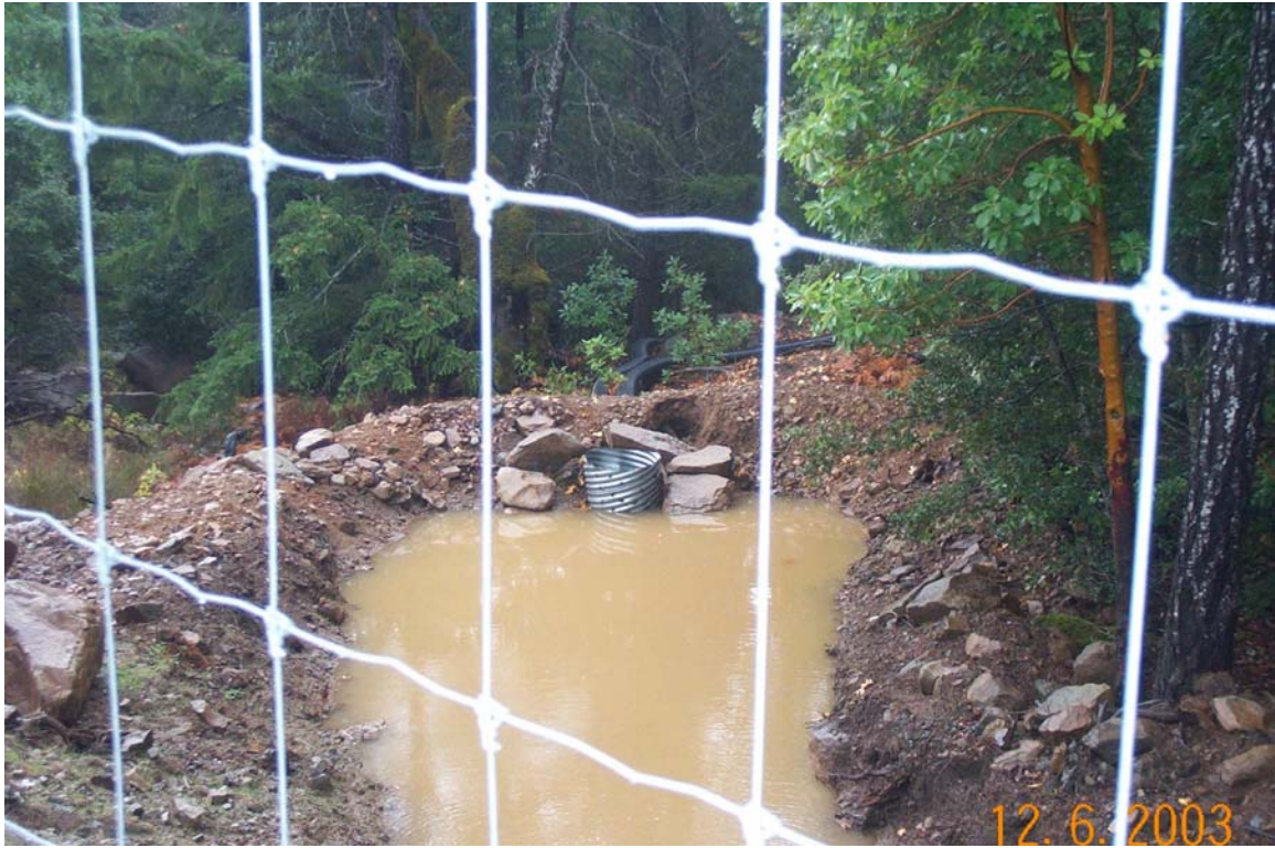
Figure 60. Sediment retention basin on tributary D12 to NF Mud Springs Creek, constructed in summer 2003. Tributary D12 originates on cultivated land, incorporates road drains, and discharges between upper and lower sensors of turbidity monitoring Station D. Photo was taken on December 6, 2003 within a few hours of the season's first heavy rainfall. Poor construction materials and methods resulted in failure of the basin berm, as indicated by the low water level. Closer examination shows piping failure along the right side of the outlet pipe, behind the large stones. This basin was not repaired during the 2003-04 runoff season, nor during summer-fall 2004. It was last observed on October 25, remaining un-repaired.
