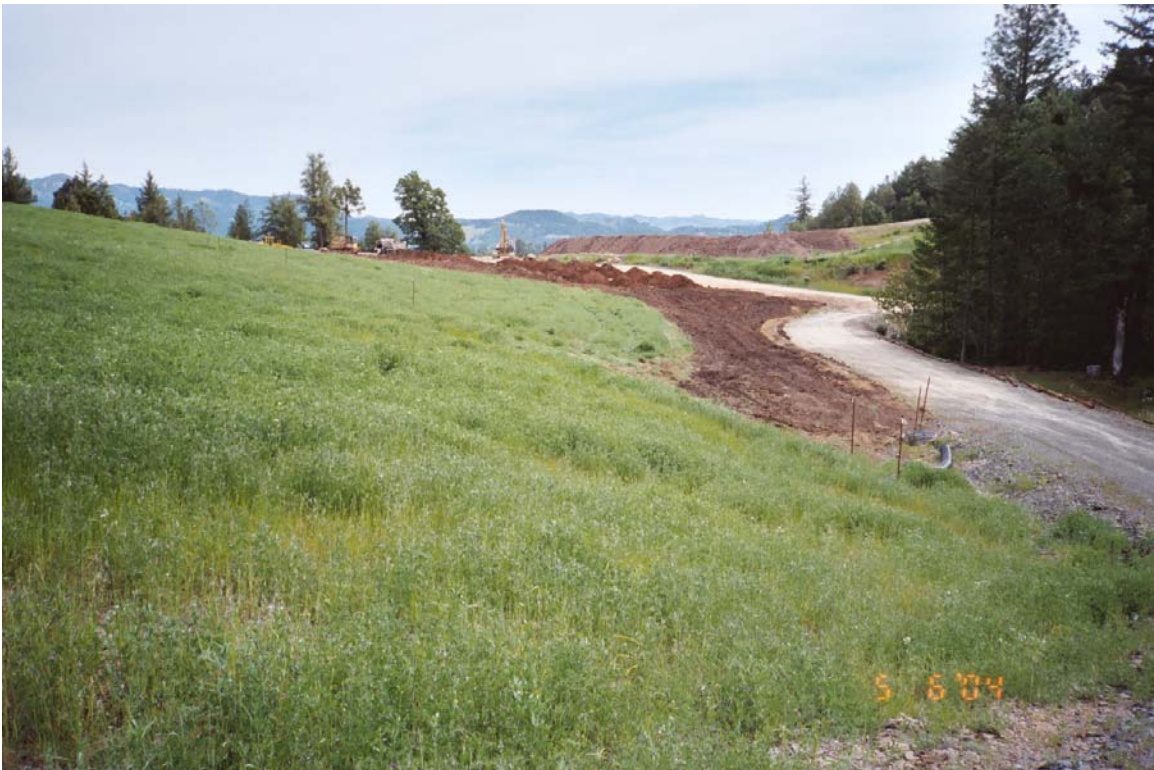
Figure 10. Fill and preparation for planting in May 2004 of an area that previously functioned as a sediment retention basin. We observed the basin acting as intended during the previous two winters by trapping sediment produced from the cultivated surface.
