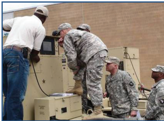
{ IT-Forward Support Base contractor instructor reviews Tactical Operations Center, or TOC, power training at a site in Iraq. }
