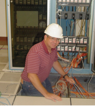
{ Eric Sundius, USAISEC IT engineer, removes old CATS and fiber optic cabling at Fort Huachuca, Ariz. }
