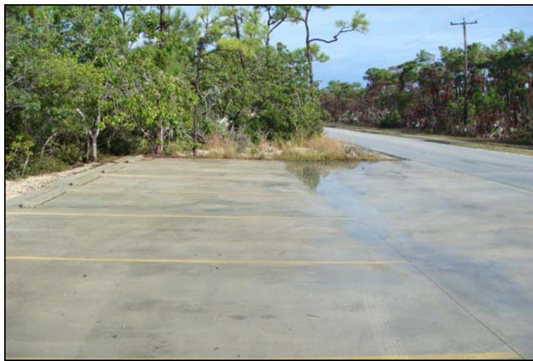
Figure 4.7: Blue Hole Interpretive Site Parking Area
