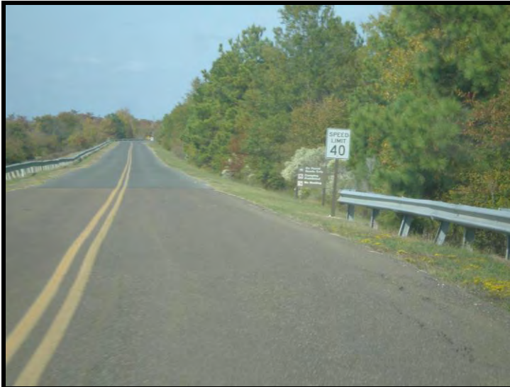
Figure 3.4: New Lock 6 Road
