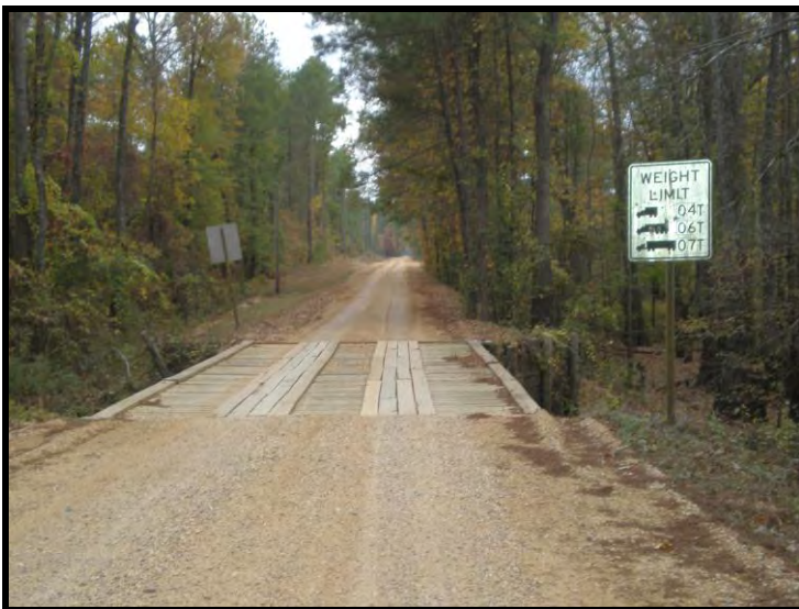
Figure 3.6: Truck restrictions on Bradley County Road 65 S Timber Bridge
