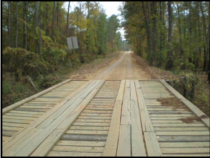
Figure 3.5: Timber bridge on Bradley County Road 65 S
