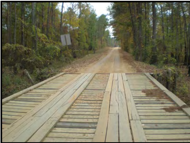
Figure 2.5: Timber bridge on Bradley County Road 65 S
