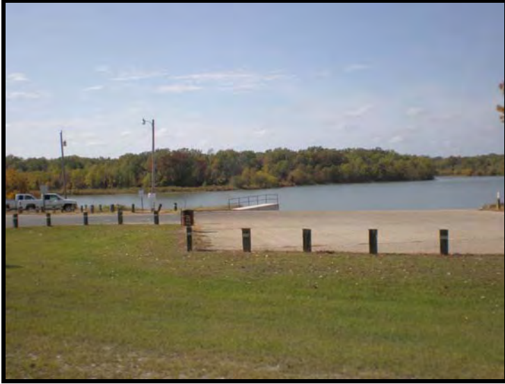
Figure 2.12: Port of Crossett Boat Ramp
