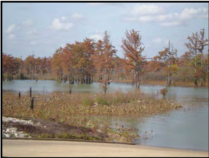
Figure 2.11: Felsenthal Lock and Dam Boat Ramp
