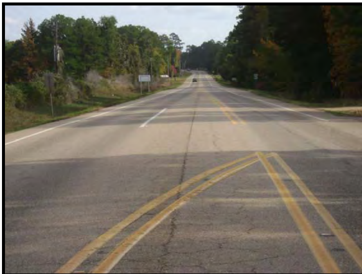
Figure 2.14: Left-Turn lane into Visitors Center
