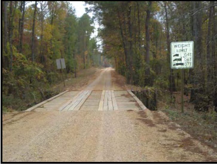
Figure 2.6: Truck restrictions on Bradley County Road 65 S Timber Bridge
