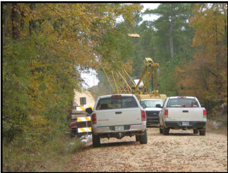
Figure 2.7: Bradley County Road 53
