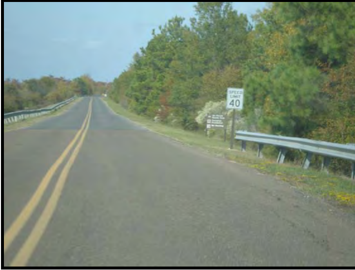
Figure 2.4: New Lock 6 Road
