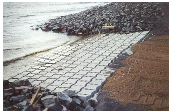
Example of block mat system used for a boat launch
