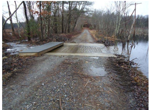
Concrete sluice on Taylor Way between two wetland areas.
