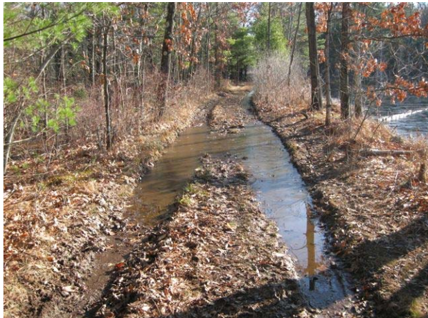
Ponding in tire ruts along Otter Alley.
