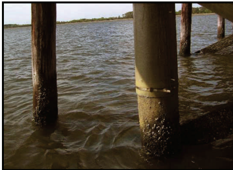
A FRP jacket is shown on the timber pile.
