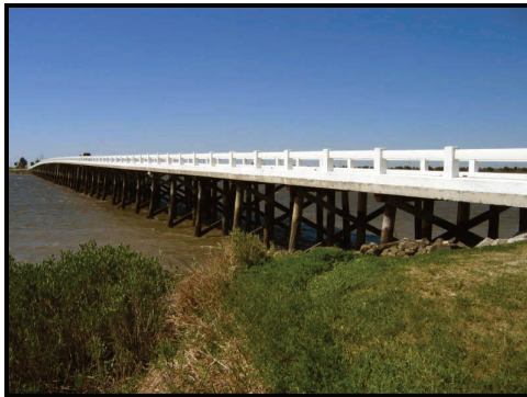
View of the bridge.
