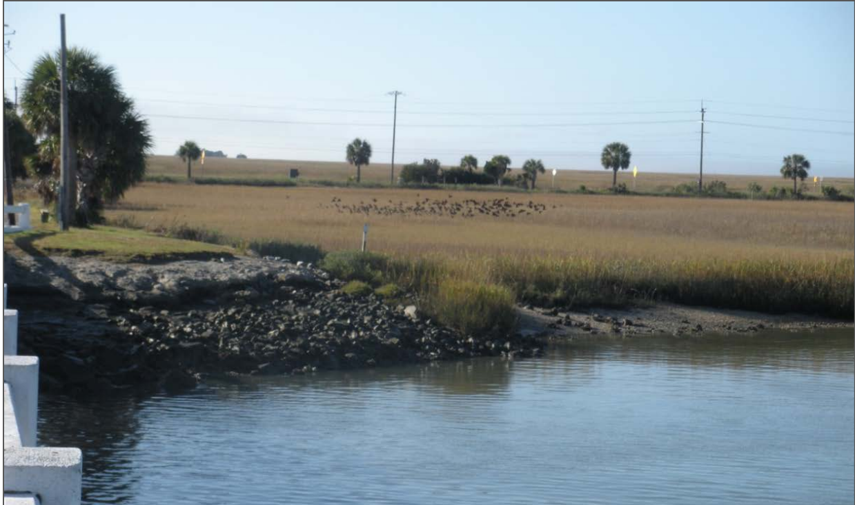
Figure 9. The tidal marsh is shown adjacent to the riprap protecting the bridge abutment.
