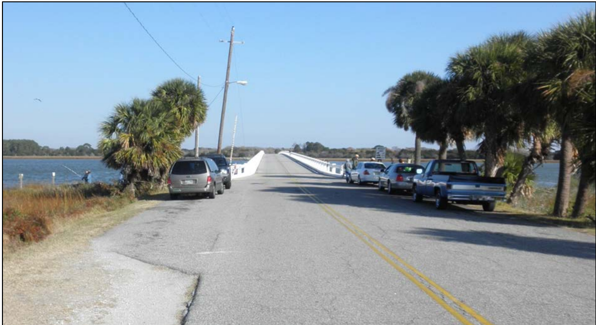
Figure 3. Two pull-offs are located on each side of the road approaching the bridge.
