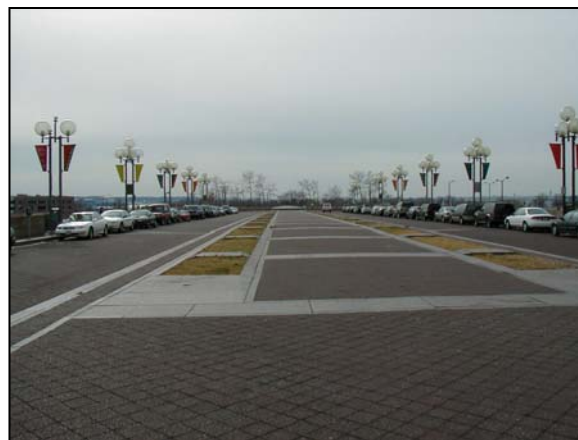
FIGURE 4-7: View from the Promenade South to the Benjamin Banneker Park Fountain
