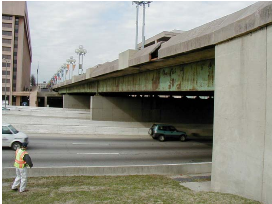
Photograph 8 L'Enfant Promenade Structure over I-395/Frontage Road.
