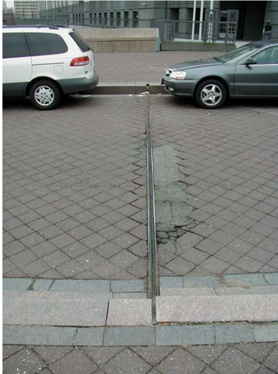
Photograph 2 Bridge No. 517, Bridge Deck.
