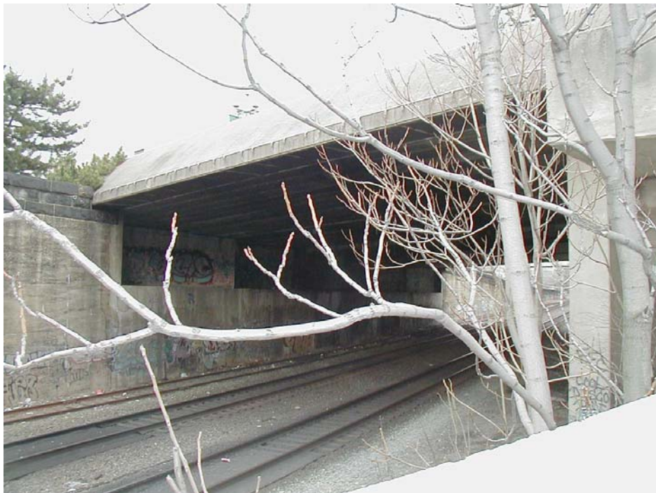
Photograph 1 L'Enfant Promenade Structure over CSX Railroad (Bridge No. 517).
