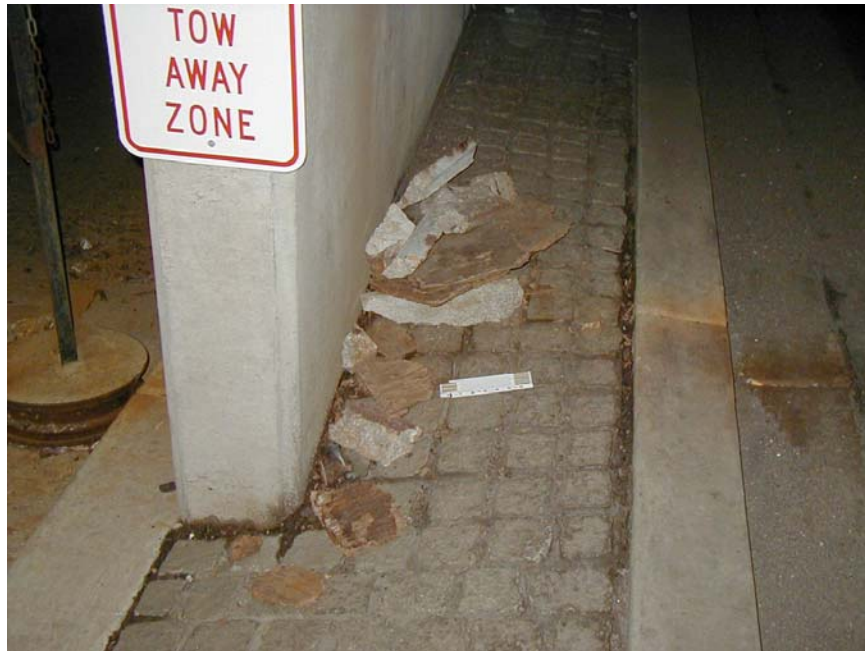
Photograph 6 Underneath Bridge No. 1114.
