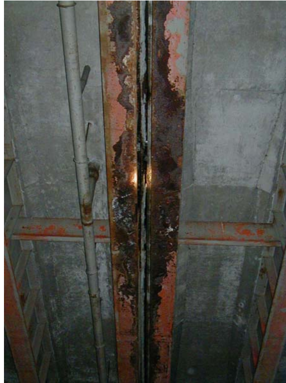
Photograph 4 Bridge No. 1114, Bridge Deck.
