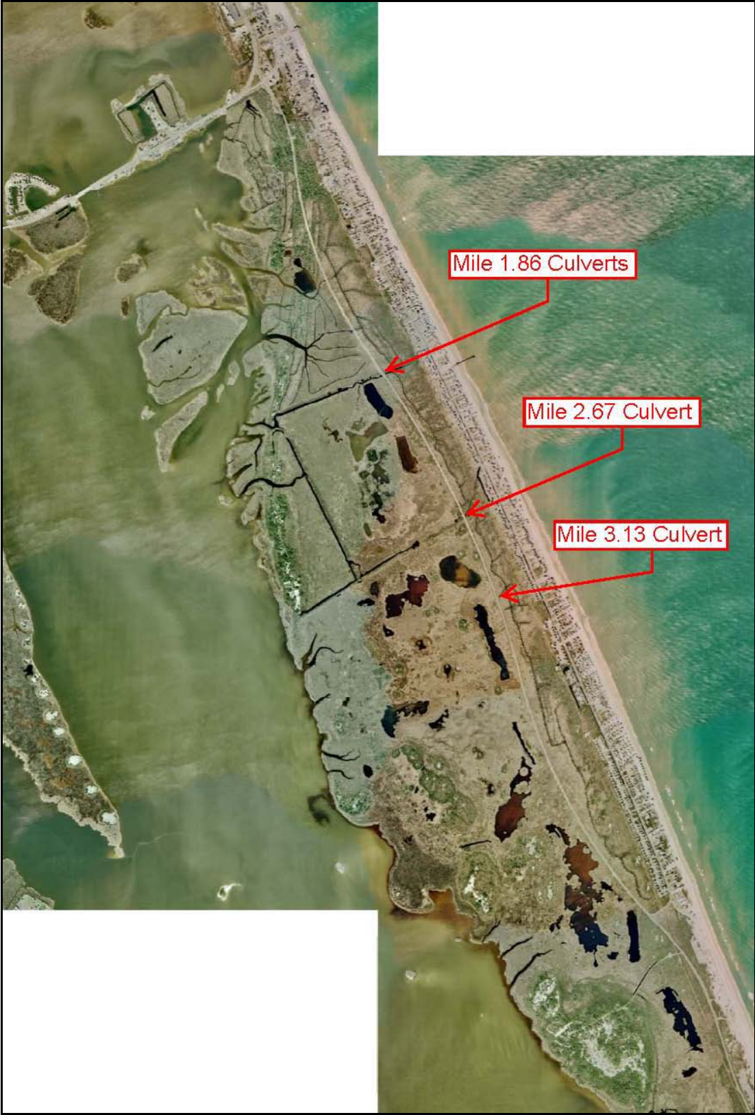
Figure 8. The three culvert replacement locations. (NC OneMap 2009)
