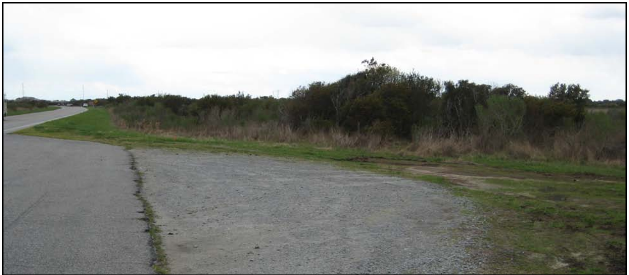
Figure 2. At this pull-off there is an additional gravel area, and rutting in the vegetated area.
