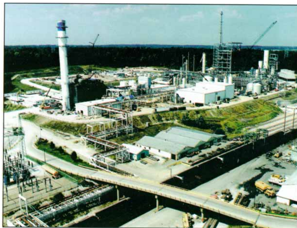
Same view as above-well into construction.
