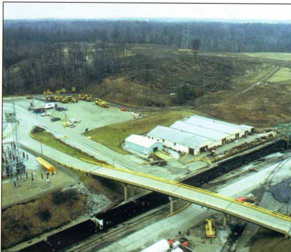
Wabash River Coal Gasification Repowering Project site during early construction.
