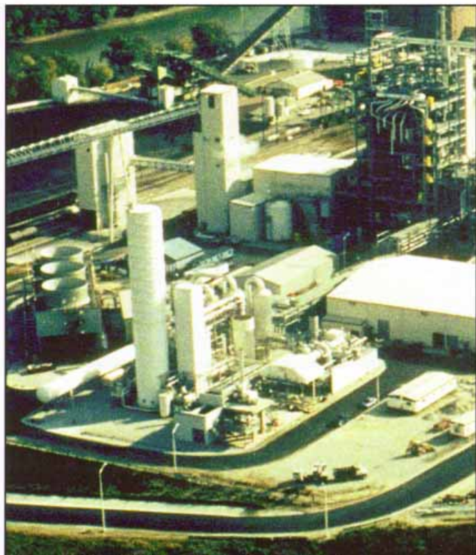
Air Separation Unit (foreground). Destec gasifier structure under construction (upper right).
