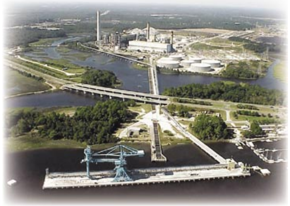
JEA plant with ship unloading dock in foreground
