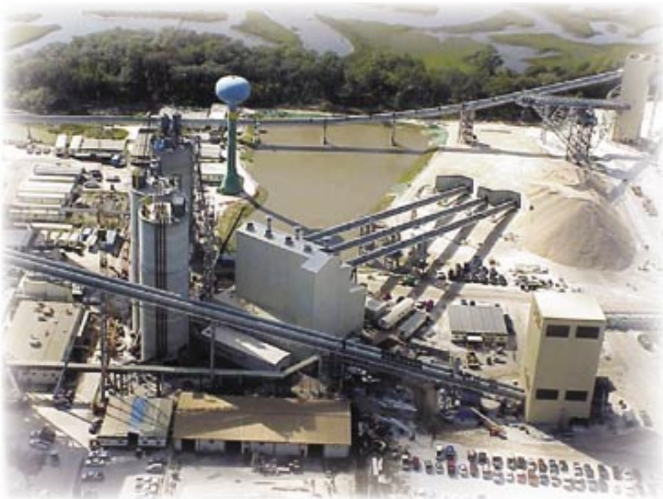
Limestone preparation system
