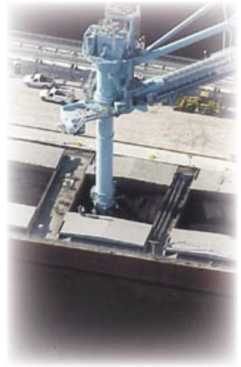
Fuel unloader at dock
