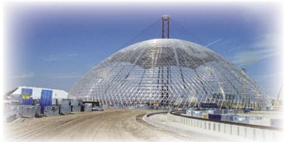
Fuel storage dome under construction
