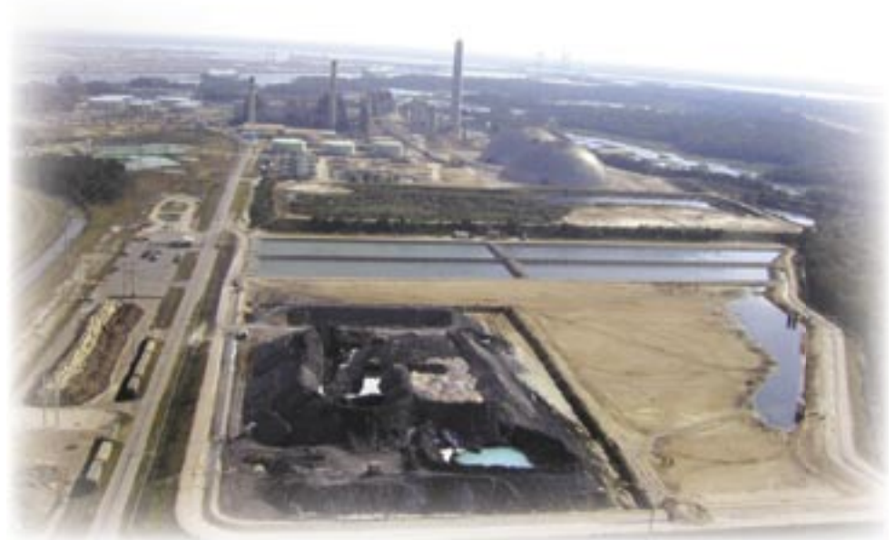
JEA plant view from by-product storage area
