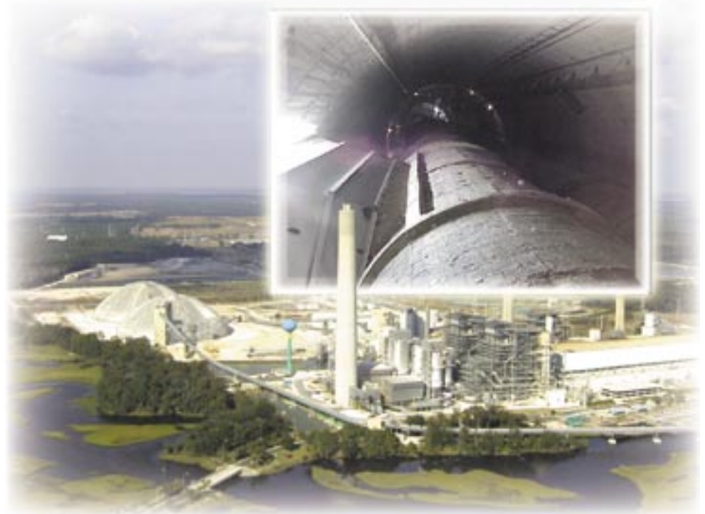
New 500-foot stack in foreground, with inset showing the stack interior
