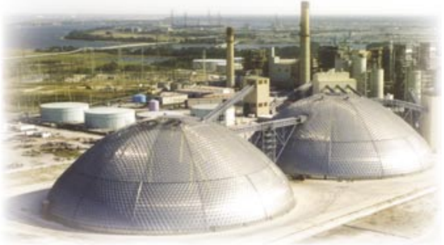
Two 400-foot diameter by 140-foot high aluminum geodesic domes for fuel storage
