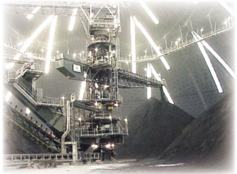
Interior of fuel storage dome
