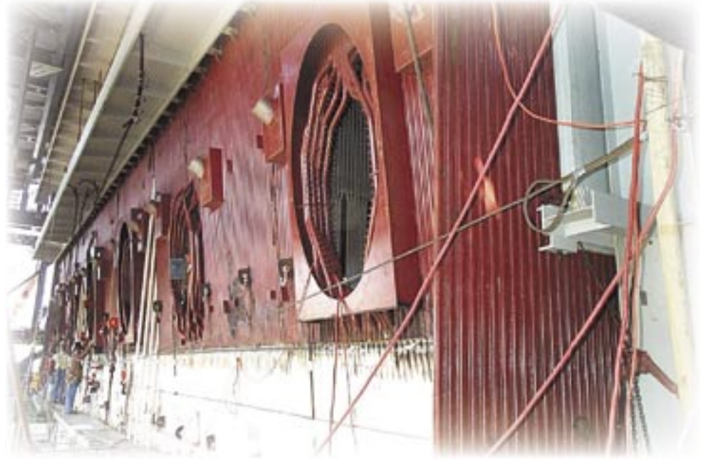
CFB boiler under construction
