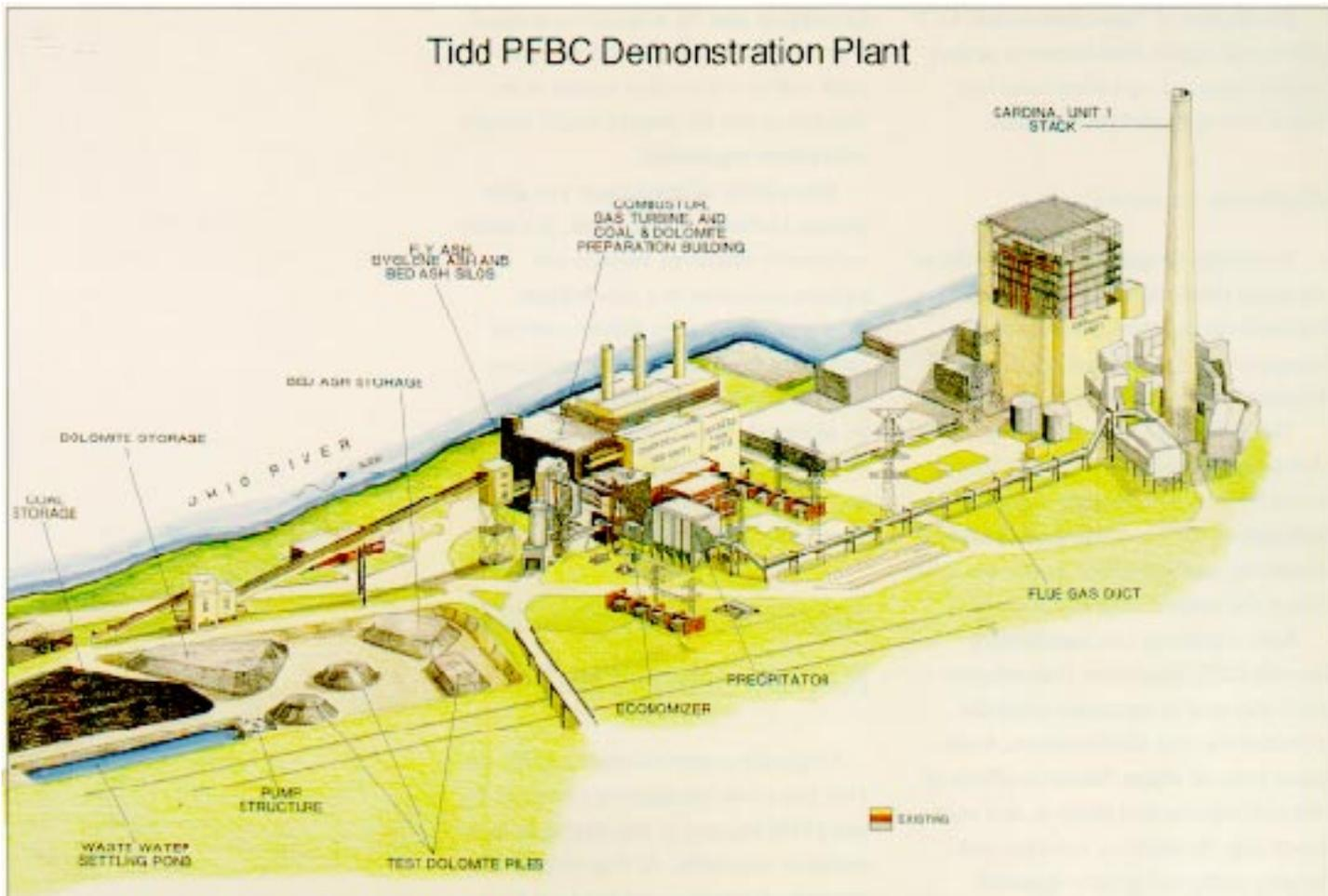
Many existing facilities at Tidd are being refurbished and reused, such as the steam cycle, fuel storage and handling facilities, and switchyard. A new building adjacent to Tidd Unit 1 houses the PFBC pressure vessel, gas turbine, and other new systems.
