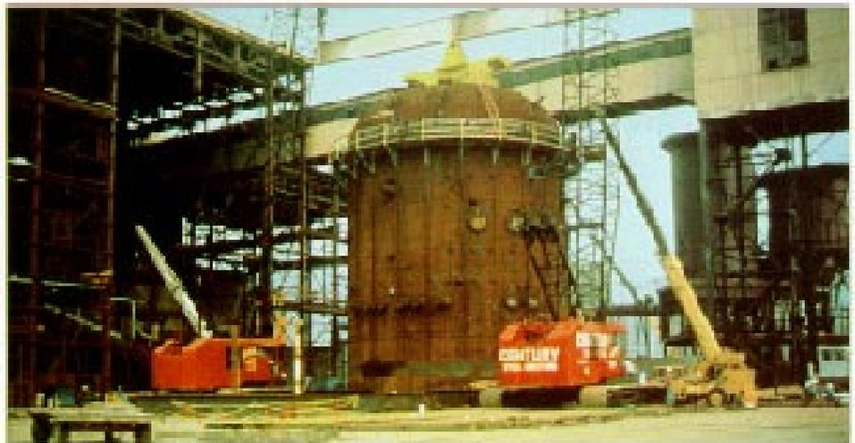
**With the barge docked at Tidd, the crew gets ready to off-load the head, detached for clearance under bridges (top). The vessel shell was moved up a 900-foot haul road, over a steel plate track laid on timber mats (center). With major internal components installed and the head repositioned, the pressure vessel is ready for the final move into the building (bottom). Once in position, the head will be arc welded in place.**
