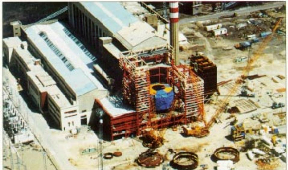
center of Stockholm. Steam from the plant will be used for district heating. The Vartan plant uses two P200 PFBC modules and a single steam turbine. The plant will have a net output of 135 MWe of electricity and more than 225 MWt of heat— while meeting extremely stringent emissions requirements. Low-sulfur (1% or less) coal will be burned; and Swedish dolomite or limestone will be used as the sorbent.
