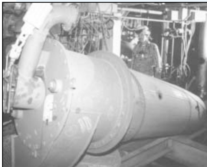
FWEC LNB installation
