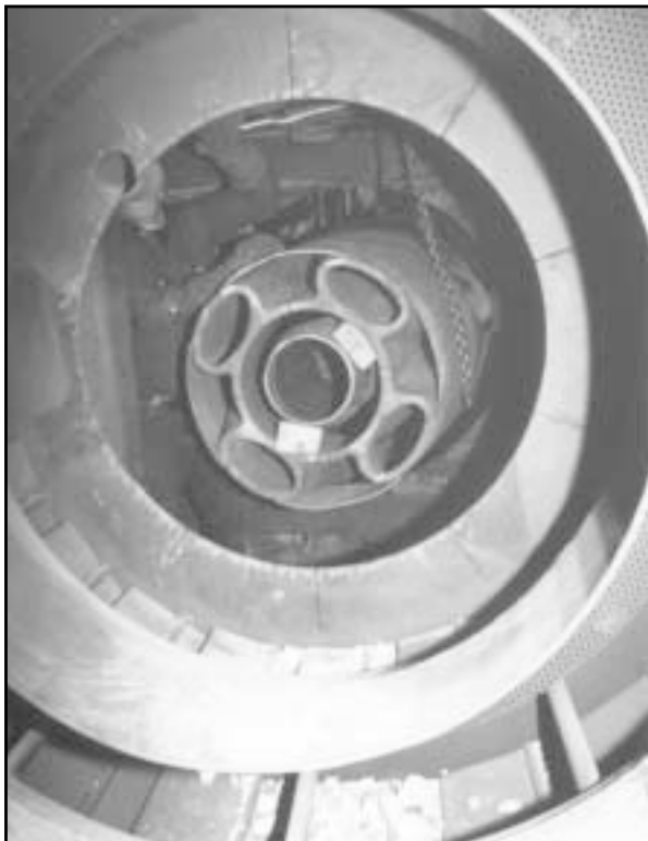
FWEC LNB showing split flame channels
