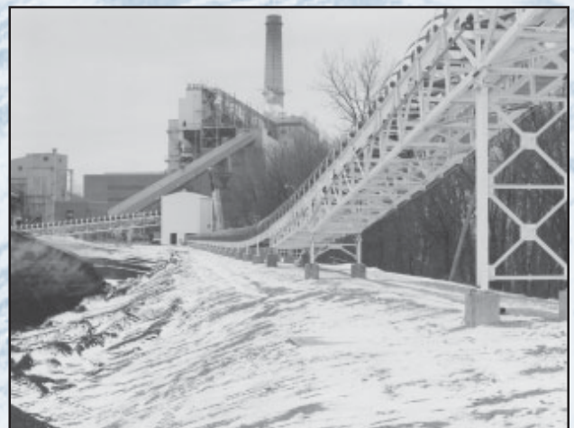
Coal receiving and handling area
