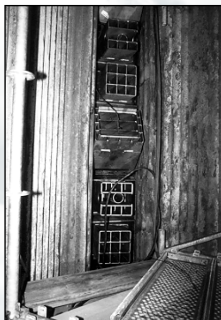
Air Injection Nozzles Top and Bottom (With Oil Guns in Two of Them) and Coal Injection Nozzle in Middle
