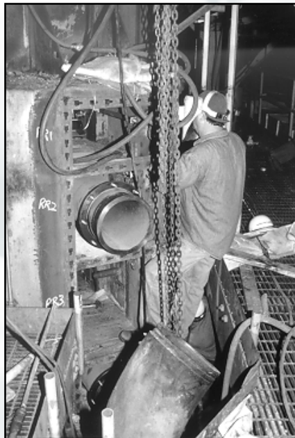
Workman Installing Coal Injection Nozzle in Corner Housing
