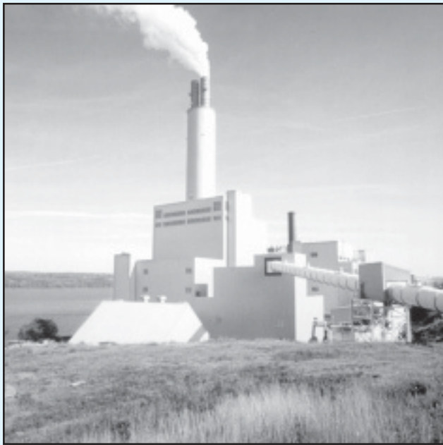
The S-H-U absorber is located beneath the stack, which saves space for plants that have space constraints.
