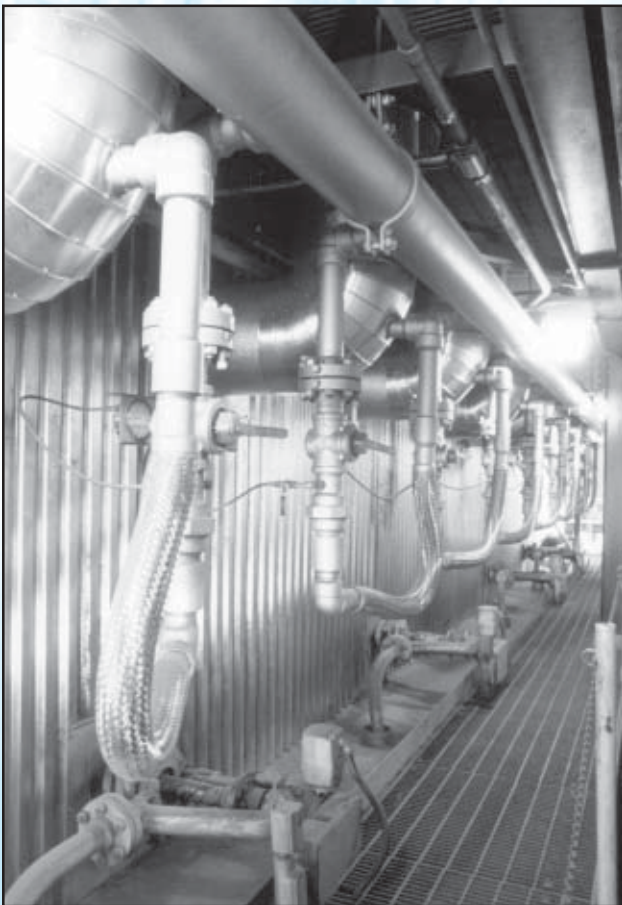
Natural gas injection system with eight injectors each on both the front and rear walls
