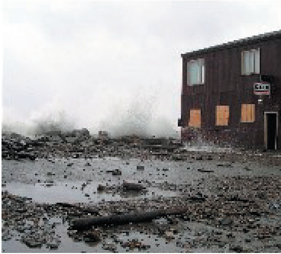
A fall storm pushes waves over the sea wall
