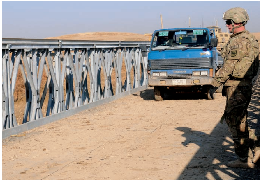
A vehicle passes over Tucker's Crossing on Jan. 27, 2012, in Helmand province, Afghanistan, constructed by members of the SDARNG's 200th Engineer Co.
