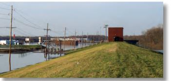
Flooding in Harrisburg, Illinois. Flooding was because of local drainage interior to the levee (foreground) that could not be evacuated quick enough by the pumping station located in the brick structure atop the levee. Photograph by Robert Holmes, USGS.
