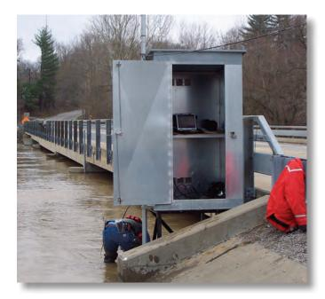
Hydrographer working to repair instrumentation on the Big Muddy River at Murphysboro, Illinois (USGS streamgage 05599490). Photograph by Robert Holmes, USGS.
