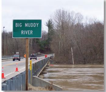
Hydrographer making a streamflow measurement on the Big Muddy at Murphysboro, Illinois (USGS streamgage 05599490). Photograph by Robert Holmes, USGS.
