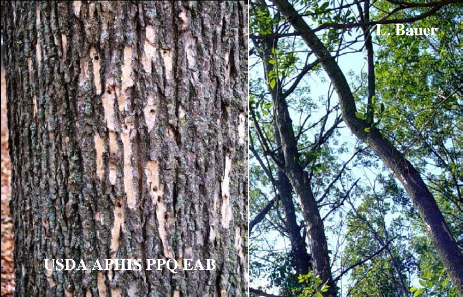
Damage from Woodpecker Feeding
