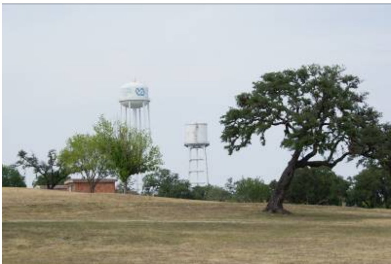
View of water towers, facing north from EUL parcel.
