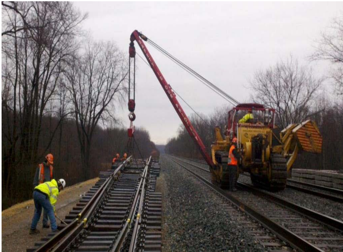
Construction of the Kent Interlocking (OH)
