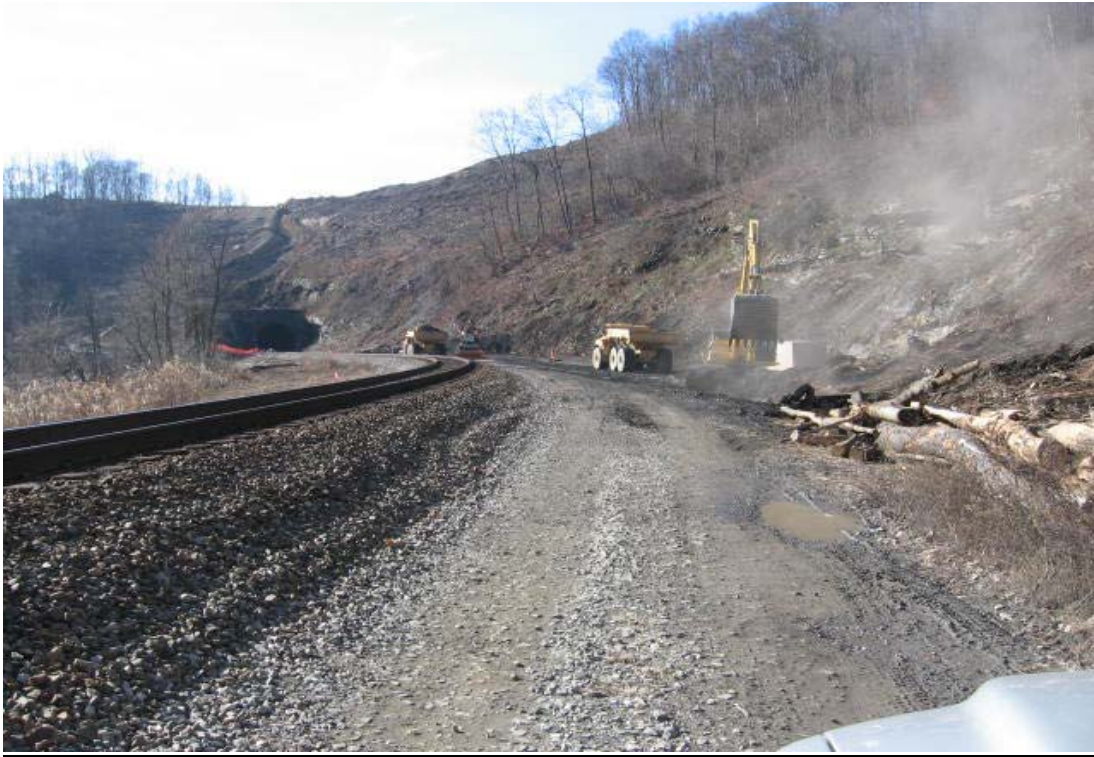
Open Cut Construction Operations at the Pinkerton Tunnel (PA)
