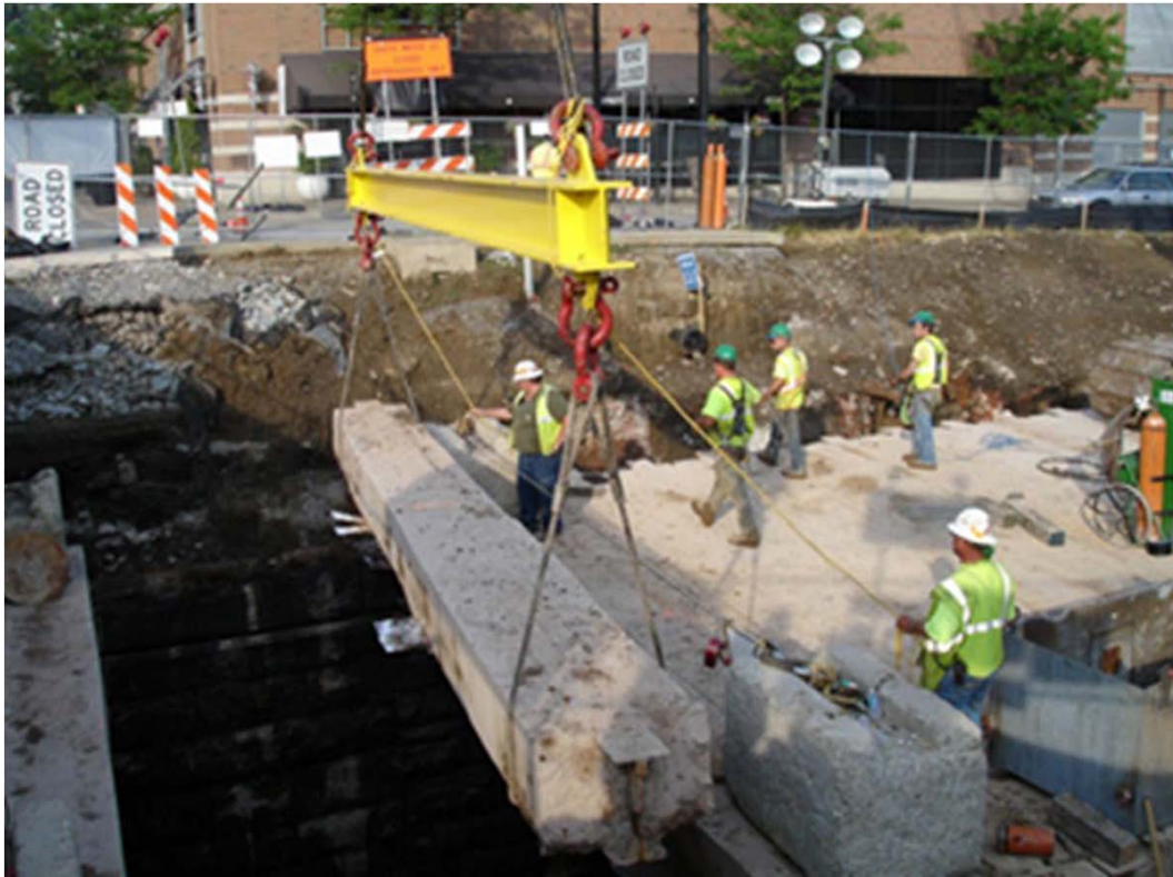
Removal of Roof Sections at J&L Tunnel (PA)
