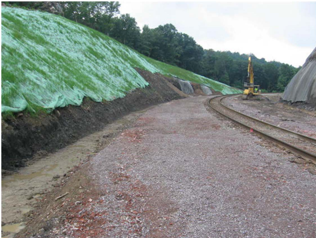
Completion of Open-Cut Operations at the Shoofly Tunnel Project (PA)
