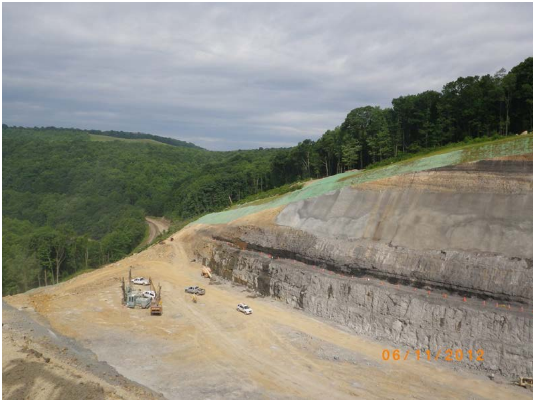
Open Cut Excavation Operations at the Pinkerton Tunnel (PA)
