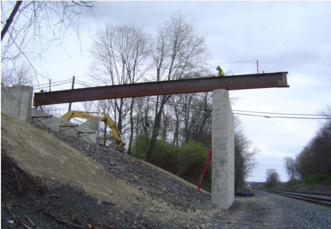
1 st Bridge Beam lifted into place at 5 th Street Project (OH)
