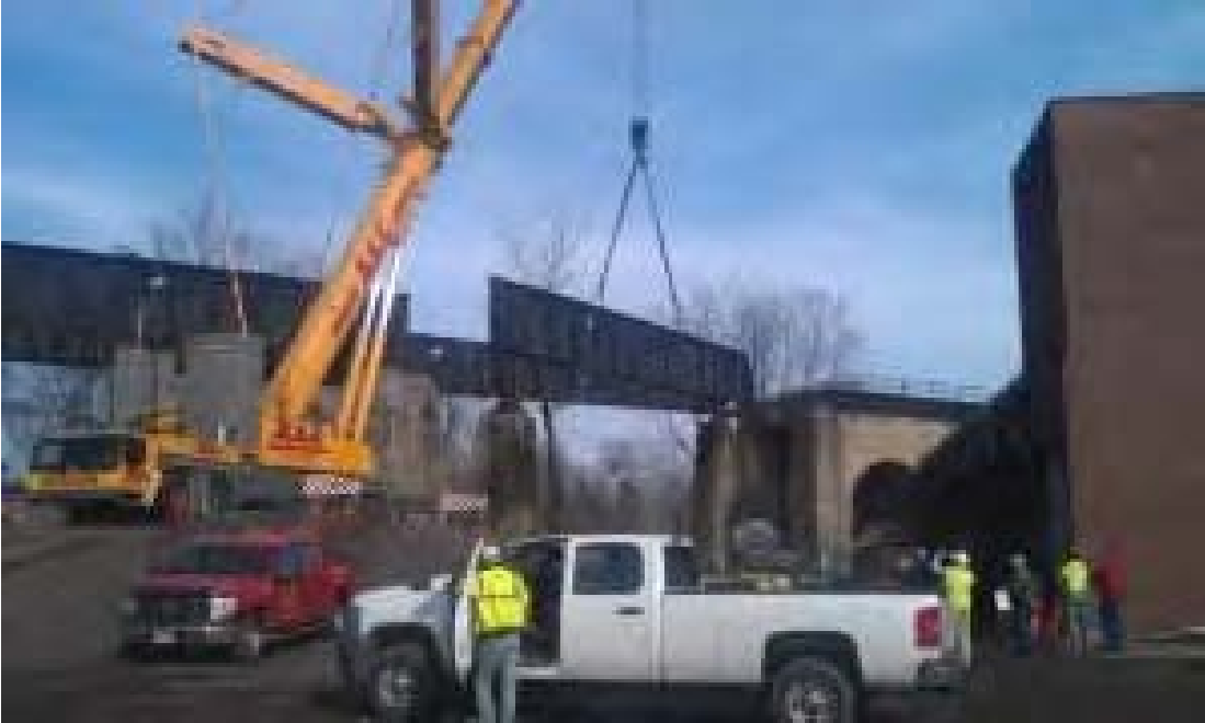
Removal of the Abandoned RR Bridge in Youngstown (OH)
