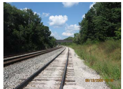
Kent W&LE Bridge Track Lowering Grade Adjustment
