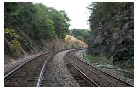
Stuart Tunnel View from East Portal
