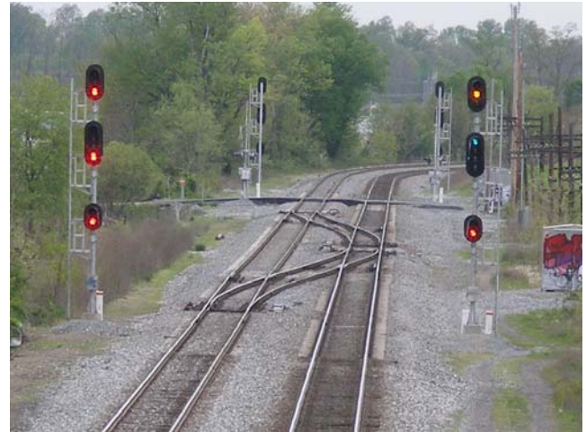
Example of Rail Interlocking
