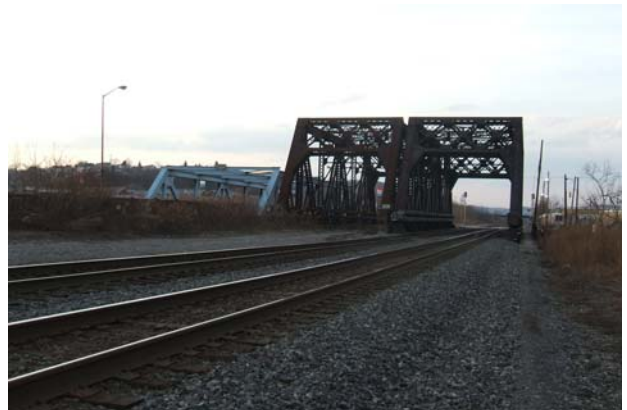
Chartiers Creek Bridge Modification
