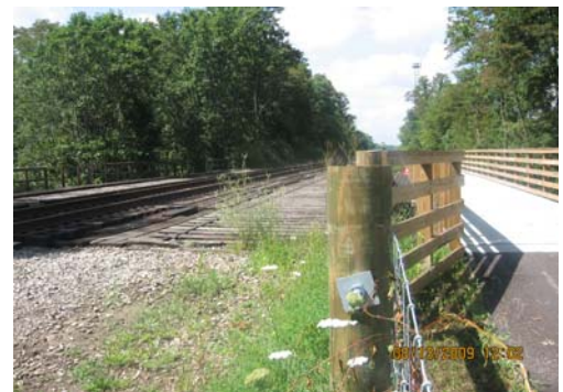
Kent Bike and Hike Trail Bridge Raising
