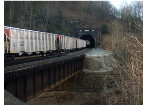
Falls Cut Tunnel
