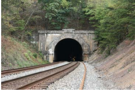
Carothers Tunnel East Portal
