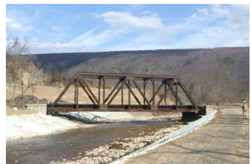
Hyndman Railroad Bridge Modification
