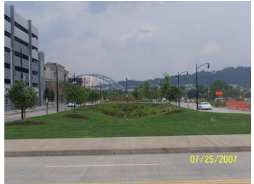
J&L Tunnel Open Space Area
