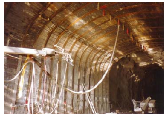
Total Arch Liner Replacement
