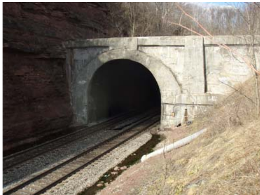
Sand Patch Tunnel Liner Notching
