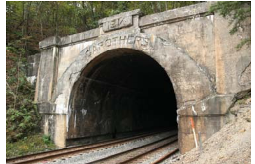
Carothers Tunnel East Portal
