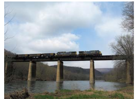
Magnolia Bridge Over Potomac River, Part of the Magnolia Cutoff
