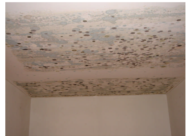
Housing Elevator Bank Hallway
