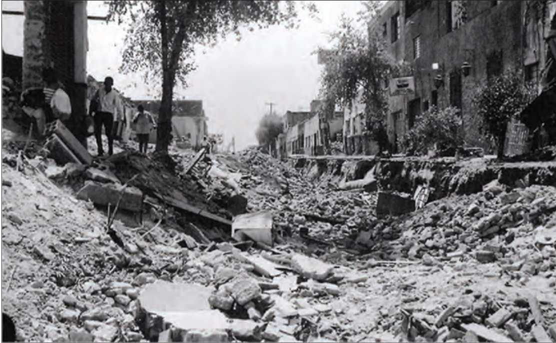
Figure 1-2. Gasoline-sewer explosion, Guadalajara, Mexico, April 22, 1992. Reprinted with permission from the Disaster Recovery Journal (Vol 5, #3).
