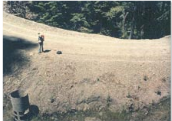
Abandoned logging road with intact culvert before treatment
