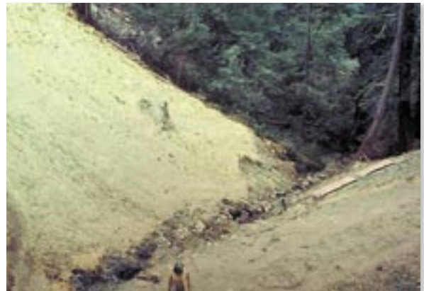
Immediately following stream-crossing excavation
