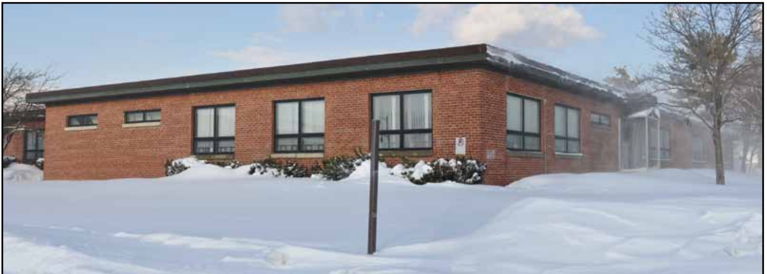
Current Air Traffic Control Squadron Operations Facilities at Pease Air National Guard Base
