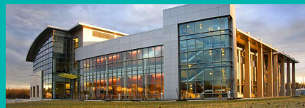
Center for Functional Nanomaterials, New York
