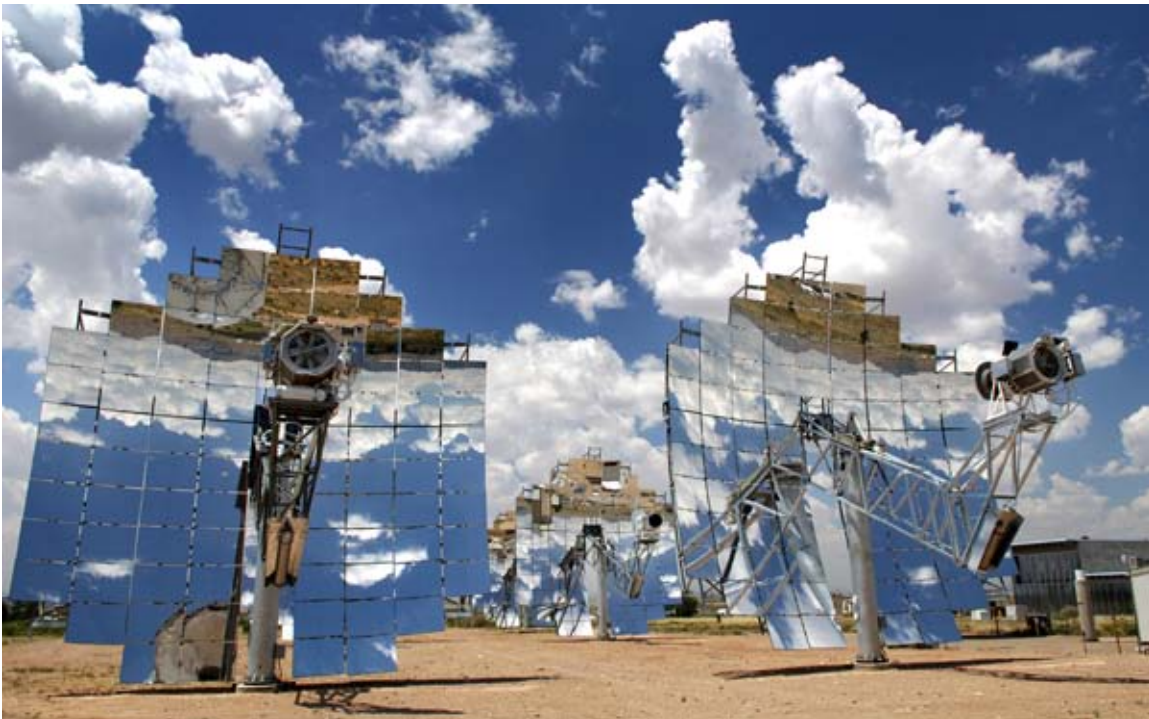
16 17 FIGURE F.2.5-1 Stirling Dish Engines at the Stirling Energy Systems Test Facility in 18 Albuquerque, New Mexico (Credit: Randy Montoya. Source: Sandia National Laboratory. 19 Available at http://www.sandia.gov/news/resources/releases/2008/solargrid.html . Accessed 20 April 16, 2008)
