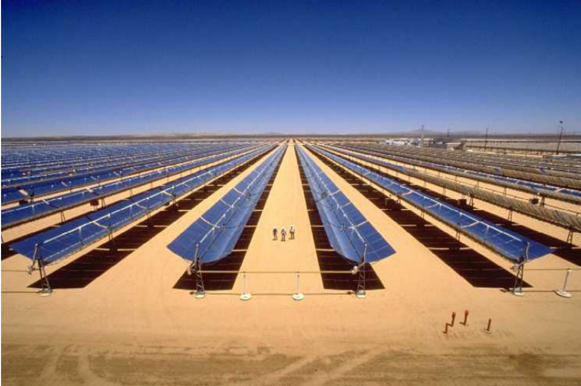
2 FIGURE F.2.2-2 Solar Field for the Florida Power and Light Parabolic Trough Facility 3 Known as SEGS VI, Kramer Junction, California (In addition to CSP, the facility also 4 includes a natural gas-fired turbine located in the facility’s power block; see background 5 right.) (Source: NREL. Available at http://www.nrel.gov/csp/troughnet/pdfs/32282.pdf . 6 Accessed June 16, 2008)
