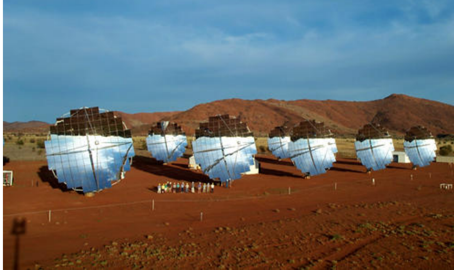
FIGURE F.3.2-5 25-kW CPV Dish at Alice Springs, Australia (The solar panels are positioned at the focal points of each of the dishes by four support arms that also serve to provide support for electrical cables and water lines for cooling jackets.) (Credit: R. McConnell. Source: NREL. Photo #13736. Available at http://www.nrel.gov/data/pix/Jpegs/13736.jpg . Accessed April 15, 2008)
