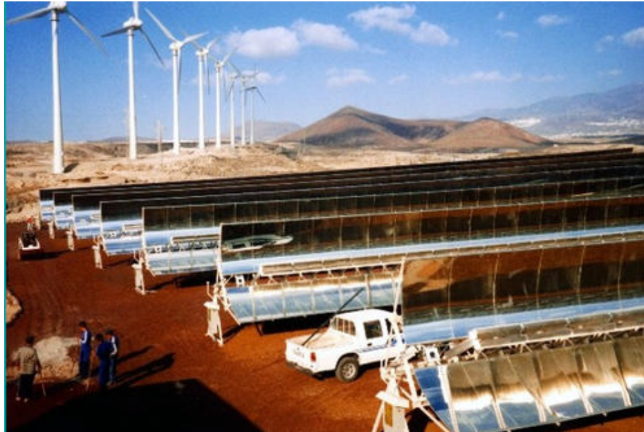
FIGURE F.3.2-6 CPV System Using Parabolic Trough Line Concentrators (This 480-kilowatt-peak (kWp) research facility is operated by the University of Madrid, Spain.) (Source: NREL. Photo #13744. Available at http://www.nrel.gov/data/pix/ . Accessed Jan. 5, 2009)
