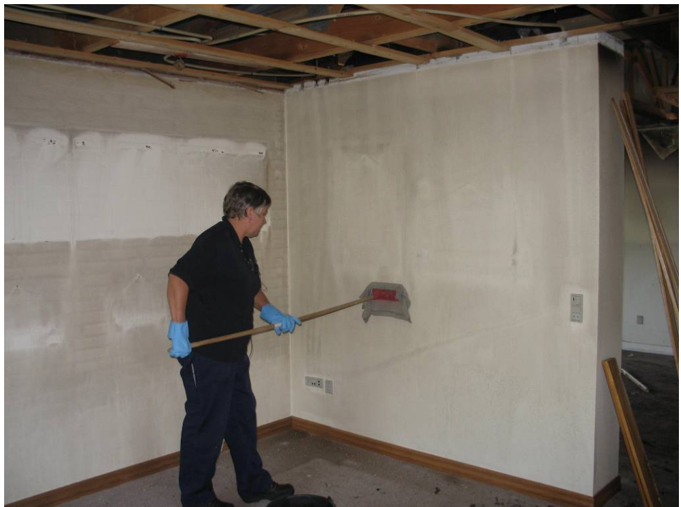
Photo 6: The stone-washed wall is being cleaned using broom and cloth.
