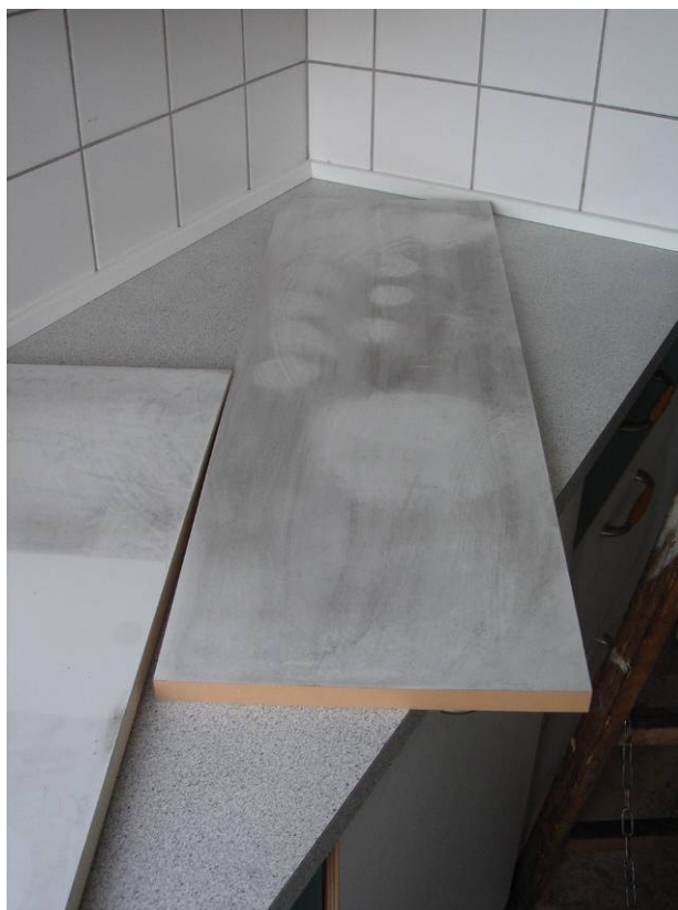
Photo 3: Soot has got in cupboards and drawers – here some loose shelves from a kitchen cupboard.
