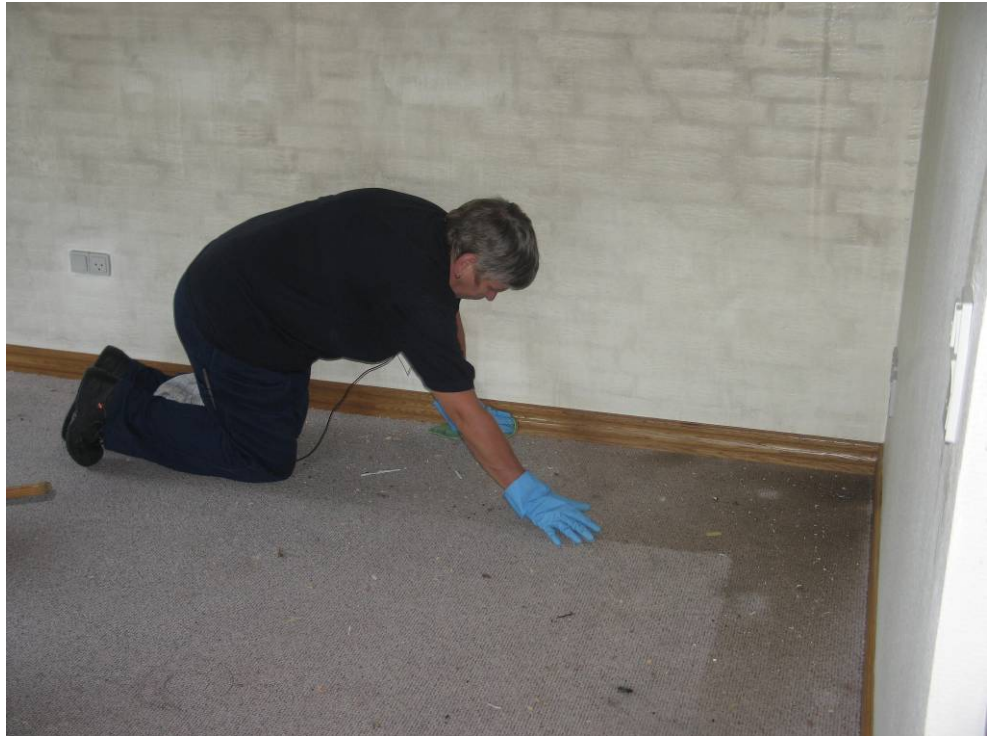
Photo 5: The skirting board is being cleaned.
