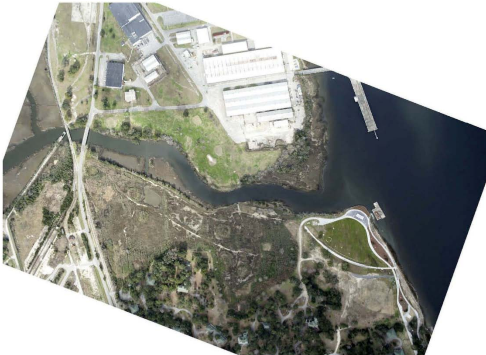
Figure 5.1 Aerial view of the Noisette Creek Project Site
