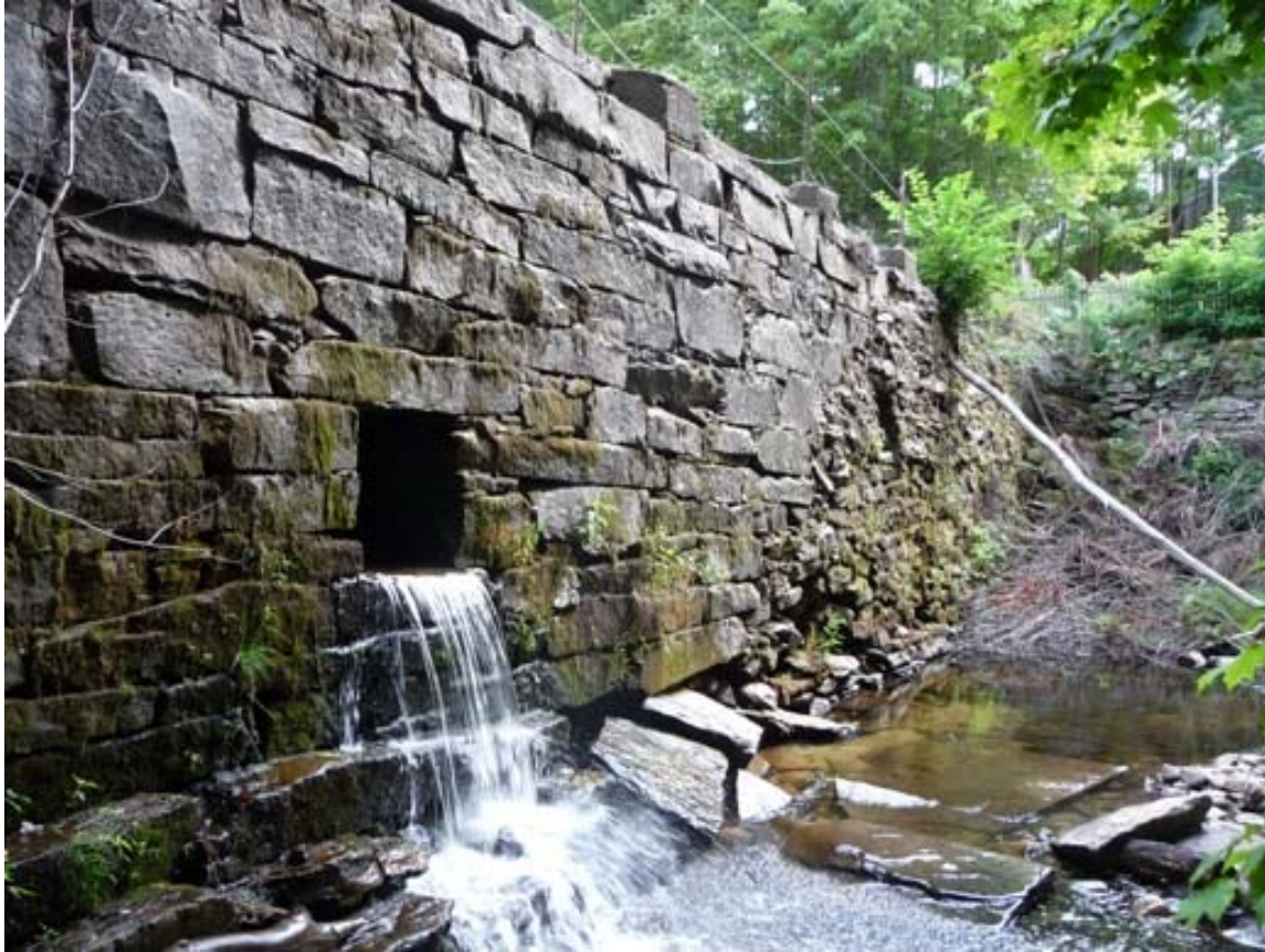
Figure 4. Downstream face of the Bartlett Rod Shop Company dam with mid-level outlet releasing Amethyst Brook flows.
