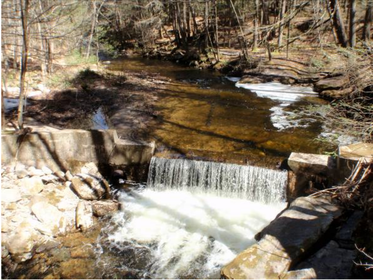
Figure 8. Orient Springs dam in Pelham, MA. Removal of this dam would provide access to spawning and rearing habitat for diadromous fish.
