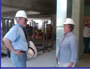
(Left) HUD officials Richard Walega, New England Regional Administrator, and Julie Fagan, Hartford Field Office Director, view construction underway at the mixed-income, mixed-use high rise complex.
