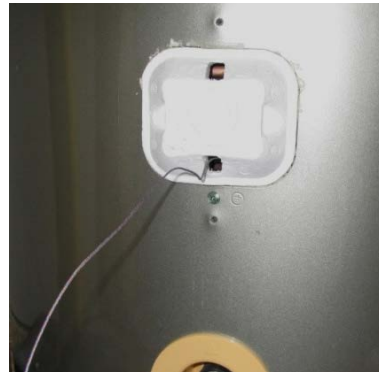
Figure 22. Insulation covering the tank where one surface-mounted TC was installed
