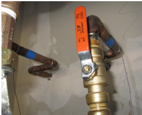
Figure 18. Surface-mounted TCs installed on the inlet and outlet water pipes
