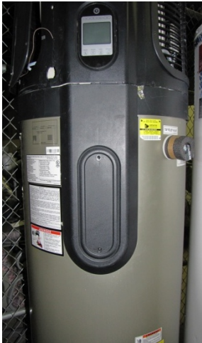
Figure 8. The A.O. Smith Voltex HPWH with the upper heater cover shown.
