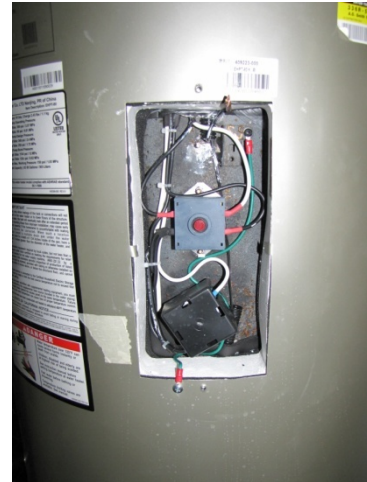
Figure 10. After the insulation is removed, the tank wall is accessible for installing a TC.
