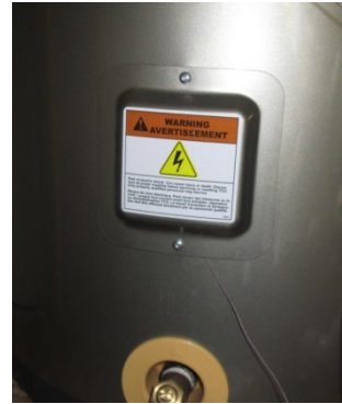
Figure 4. The cover is replaced, with the lower screw not fully tightened to give TC wire clearance.
