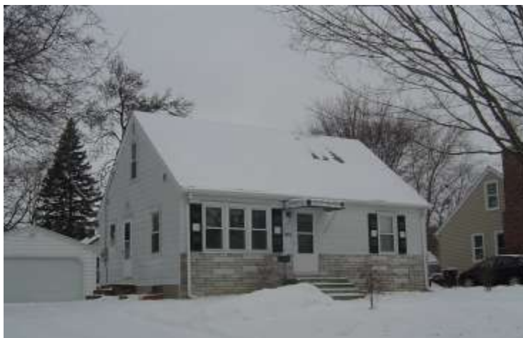
Figure 7. Typical house with two concrete stoops
