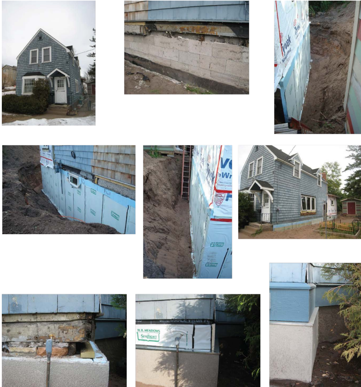
Figure 6. Full foundation excavation and insulation in Duluth
