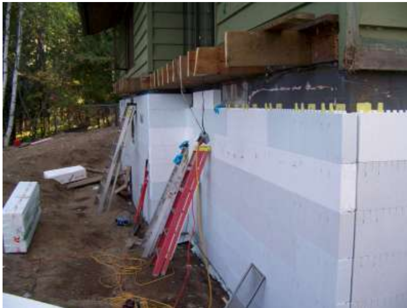
Figure 5. Installation of 4-in. EPS R-ETRO
