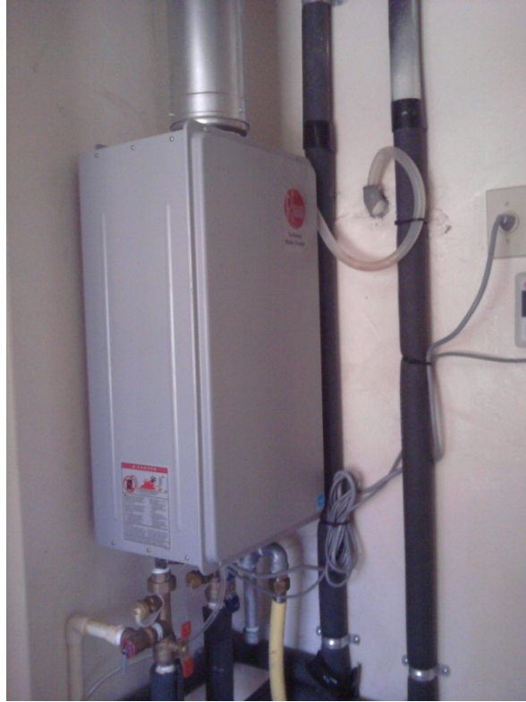
Figure L.1. Tankless hot water heater unit
